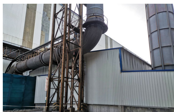
Billet line dust removal system
